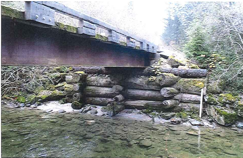
CK2109 Left Abutment
