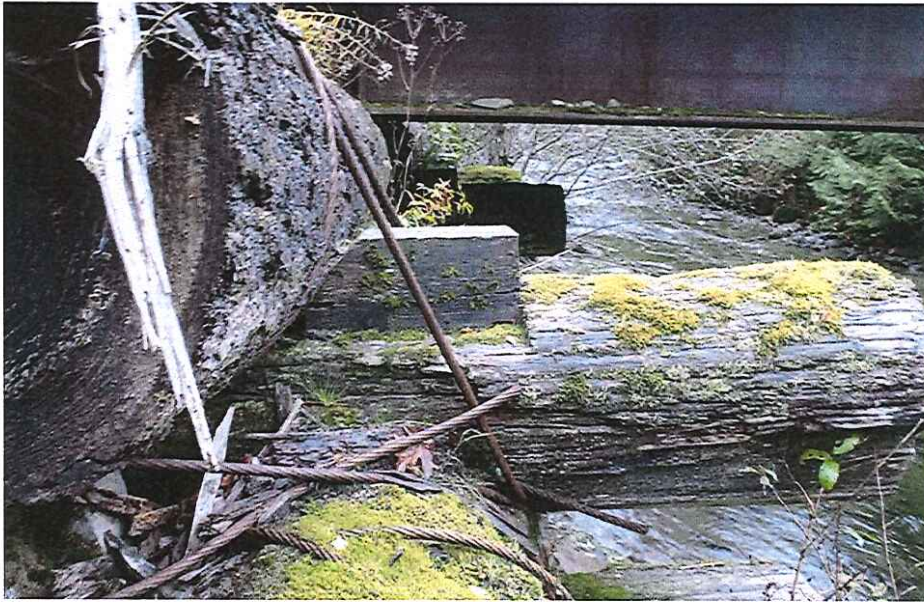
CK2109 Right Abutment
